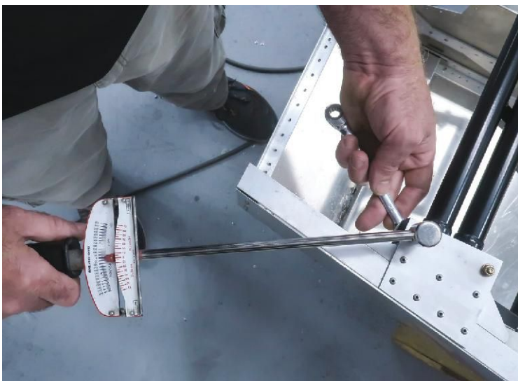
Using a beam-type torque wrench isn't always possible. If the nut in this photo had been inside the structure, instead of on top, it would limit the torque wrench's range of motion and make reading the scale impossible.
